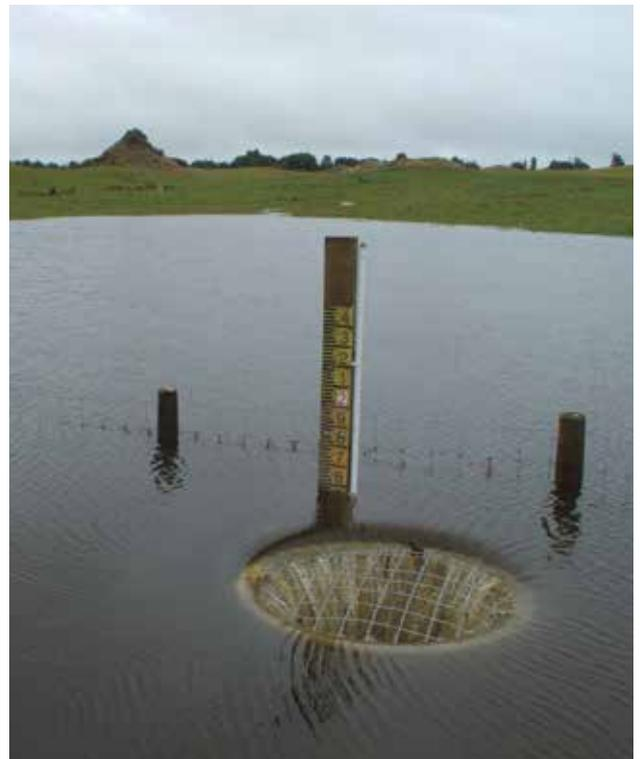
A detainment bund filled to capacity after a storm event, with stormwater leaving the bund through a riser PHOTO: John Paterson, Rotorua
