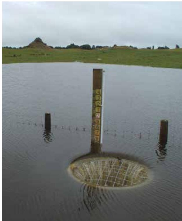
A detention bund filled to capacity after a storm event, with stormwater leaving the bund through a riser PHOTO: John Paterson, Rotorua
